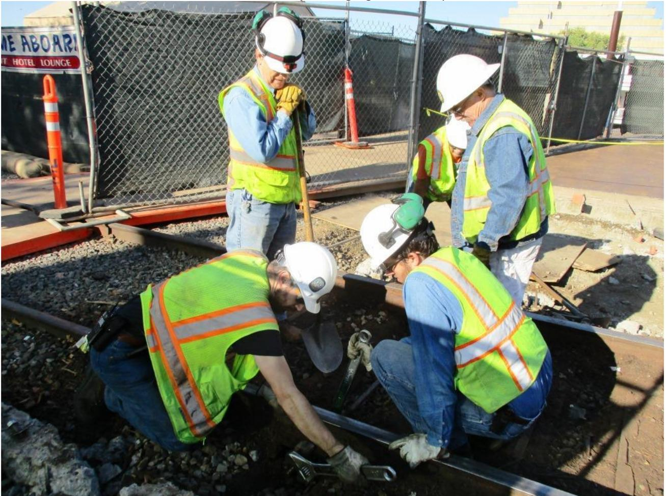
Matt and Weston tighten-down the clamps on the gauge-rod
