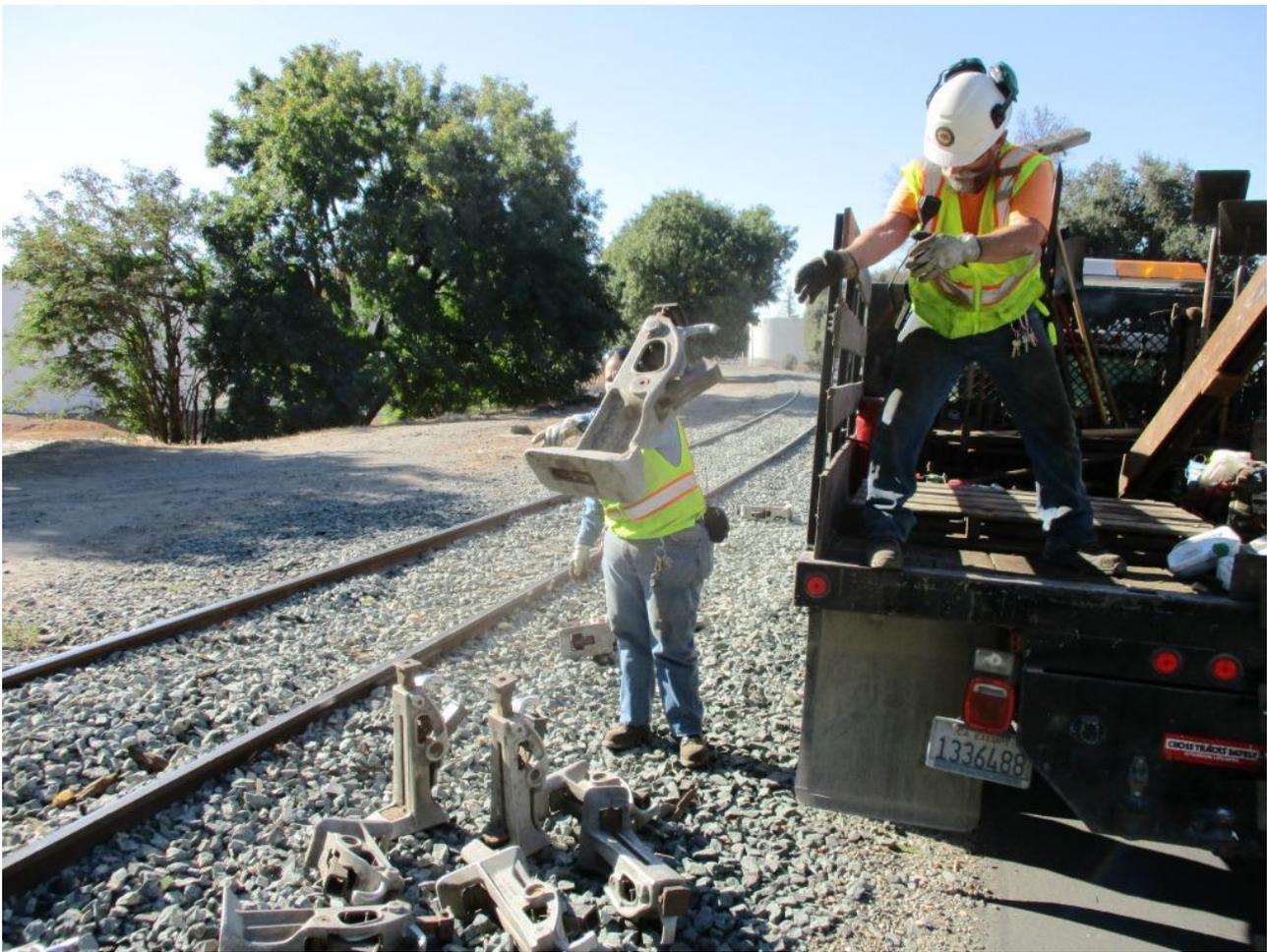
At the track-raise site, Joe deploys track-jacks from the back of the truck
