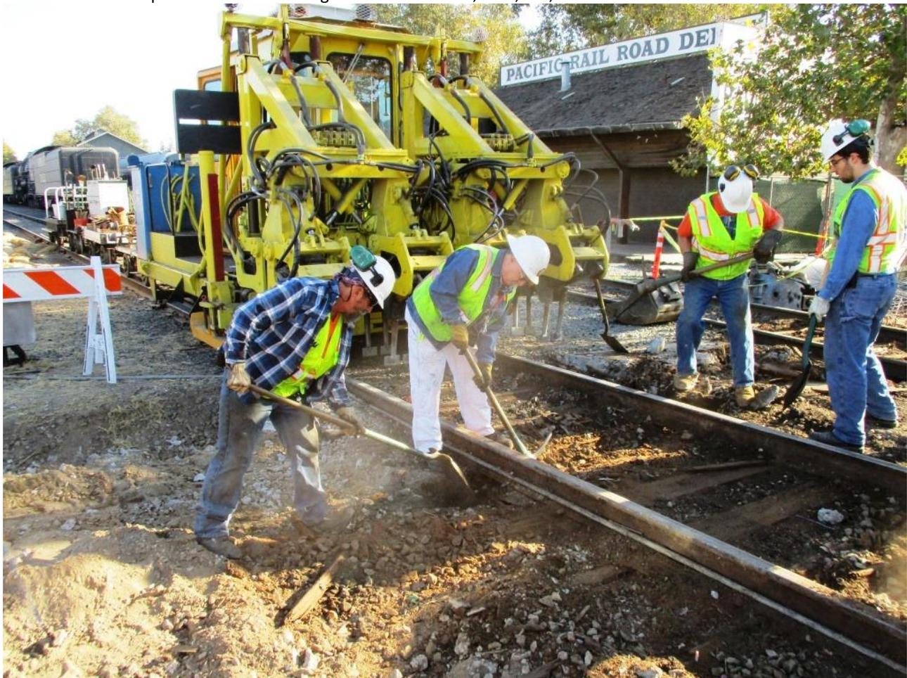
Joe, Mike H., Clem, and Weston clean-up the Old Main and dig-out pockets under the rails for the installation of gauge-rods
