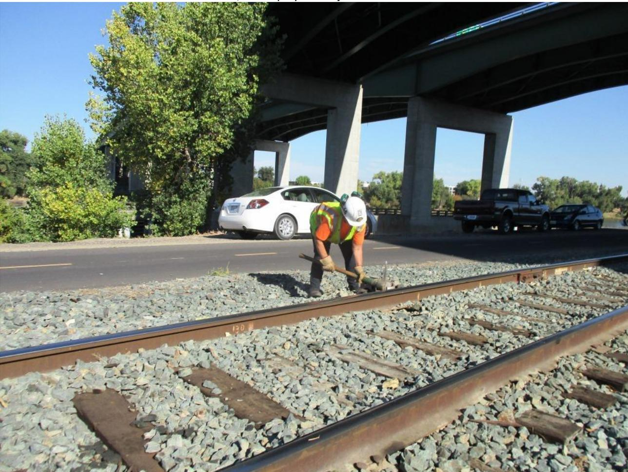
Pam gets to work digging pockets under the rail for the track-jack to be inserted
