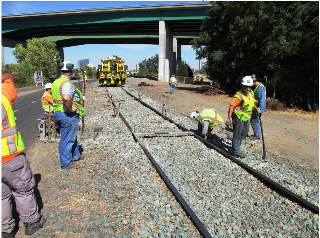
Super-elevation has been reestablished on the west rail in the curve and now we return to level as the curve straightens out
